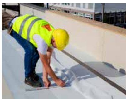
2. Mark position of upper parapet edge
