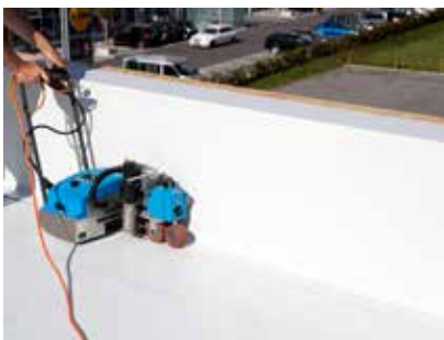
5. Final hot air seam welding
