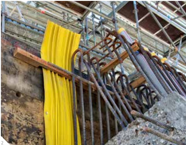
2 Sika White Box concept/Watertight concrete
