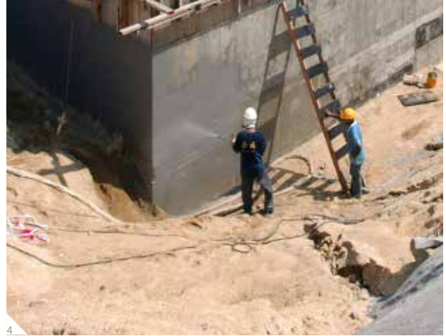
4 Liquid applied reactive membranes (PUR/PUA)
