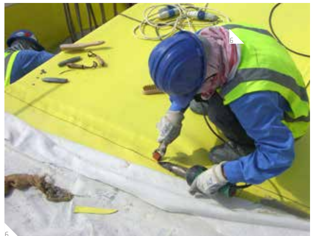
6 Compartmentalized sheet membrane systems
